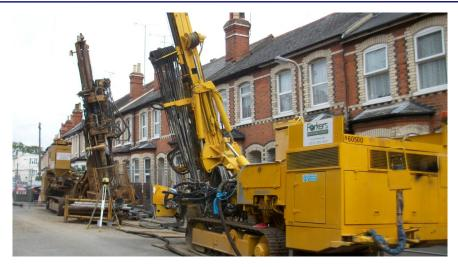
During rotary investigation drilling various parameters were recorded including rotation speeds, air pressures, penetration rates and flush returns which gave Peter Brett engineers a clear indication of ground conditions and the presence of mining anomalies.
